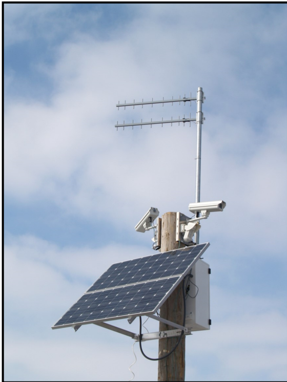
Solar Powered Video Surveillance with Motion Detection and Cellular Backhaul
