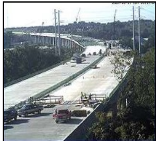
Cellular Construction Camera for Illinois Tollway Project
