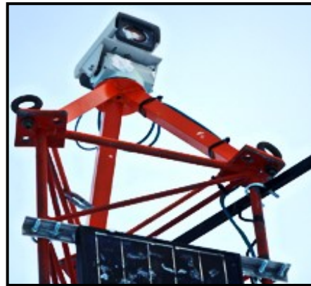
Canadian Rockies PTZ Camera for Weather and Avalanche Warning Systems
